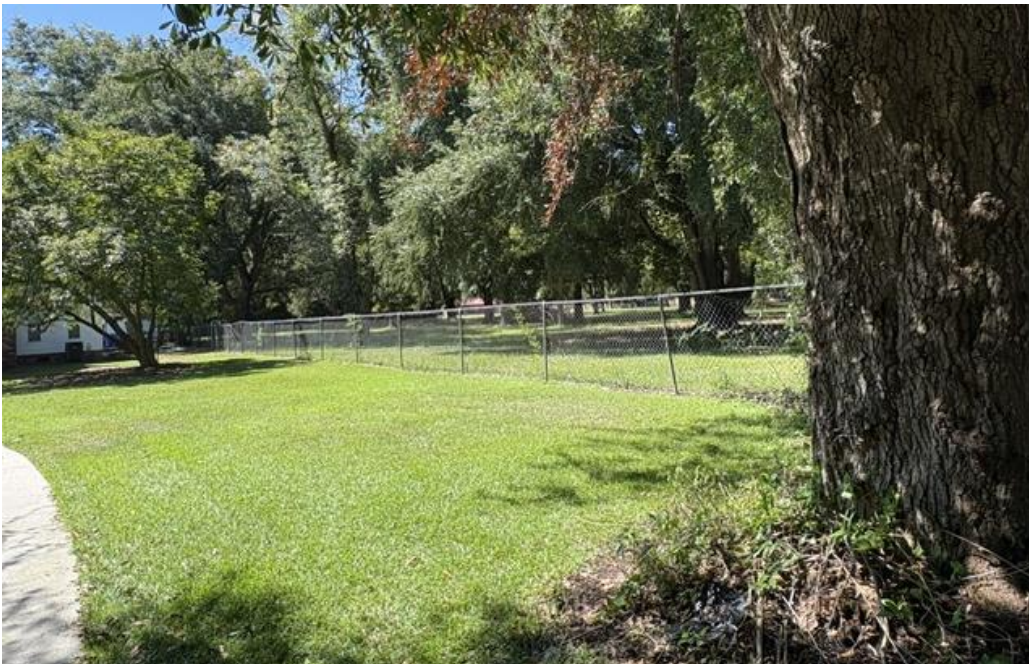
Looking down the affected side of the house from Cherokee Road and the undeveloped adjacent parcel.
