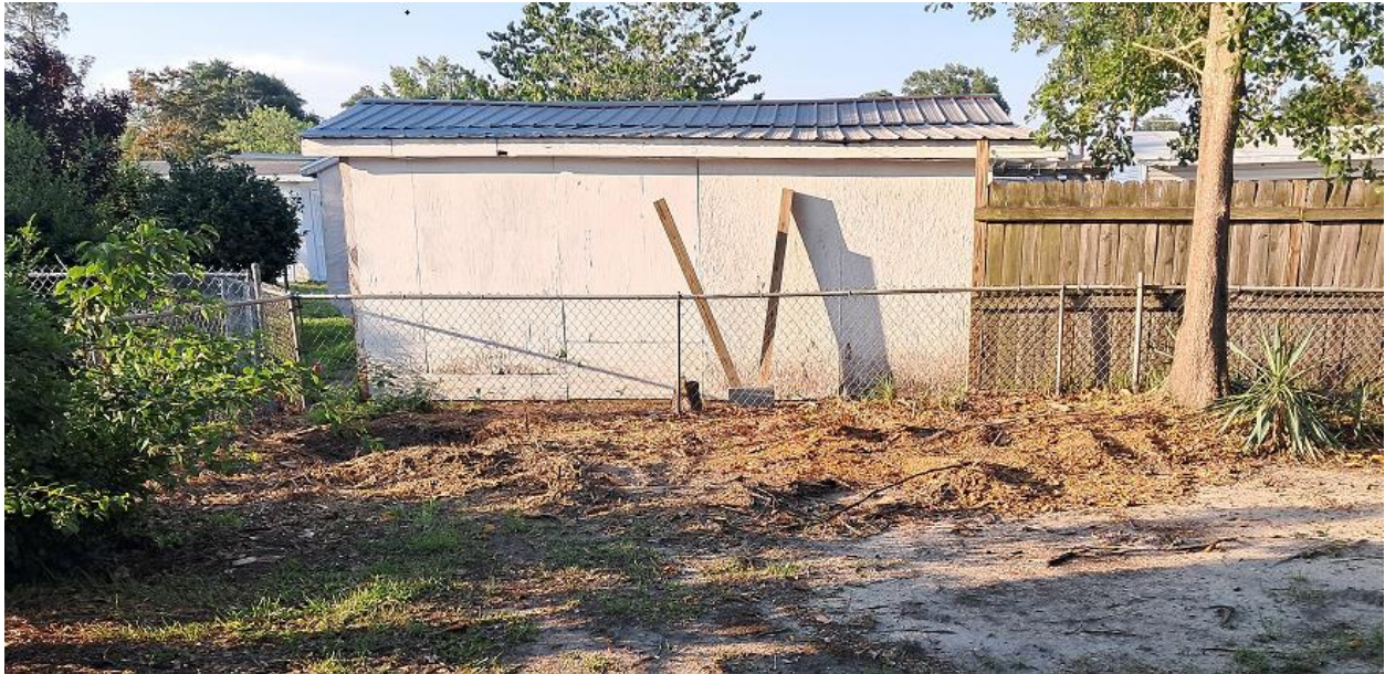
The next door neighbor's shed in proximity to the common property line.
