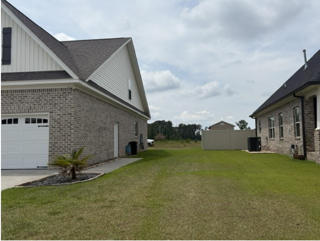
The view of the backyard from the front right side of the house.
