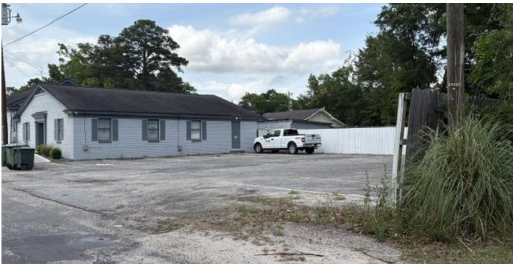
Across the street looking northeast.
