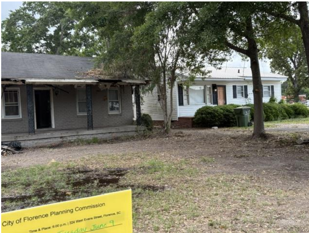
The house to the north.
