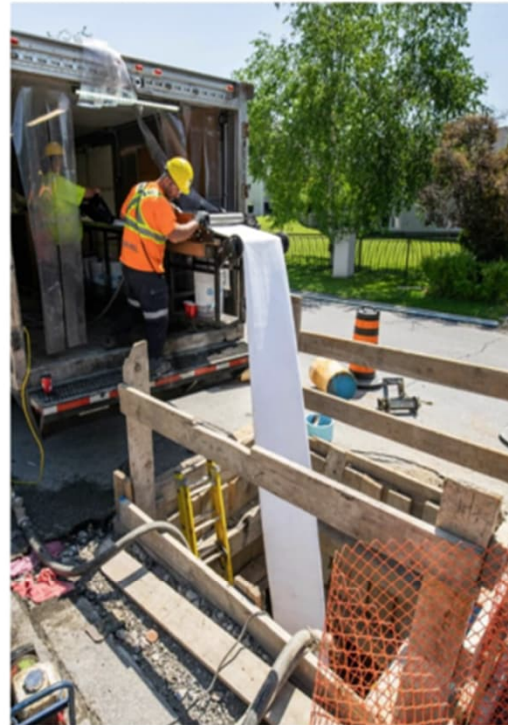
Structural Re-Lining
