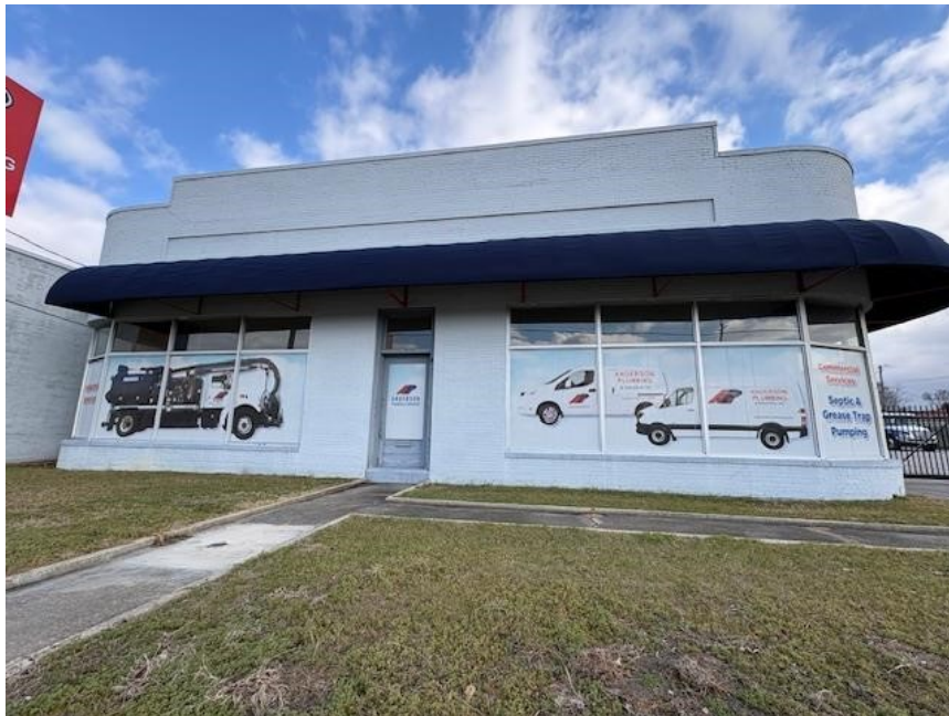
100% coverage seen from adjacent sidewalk.
