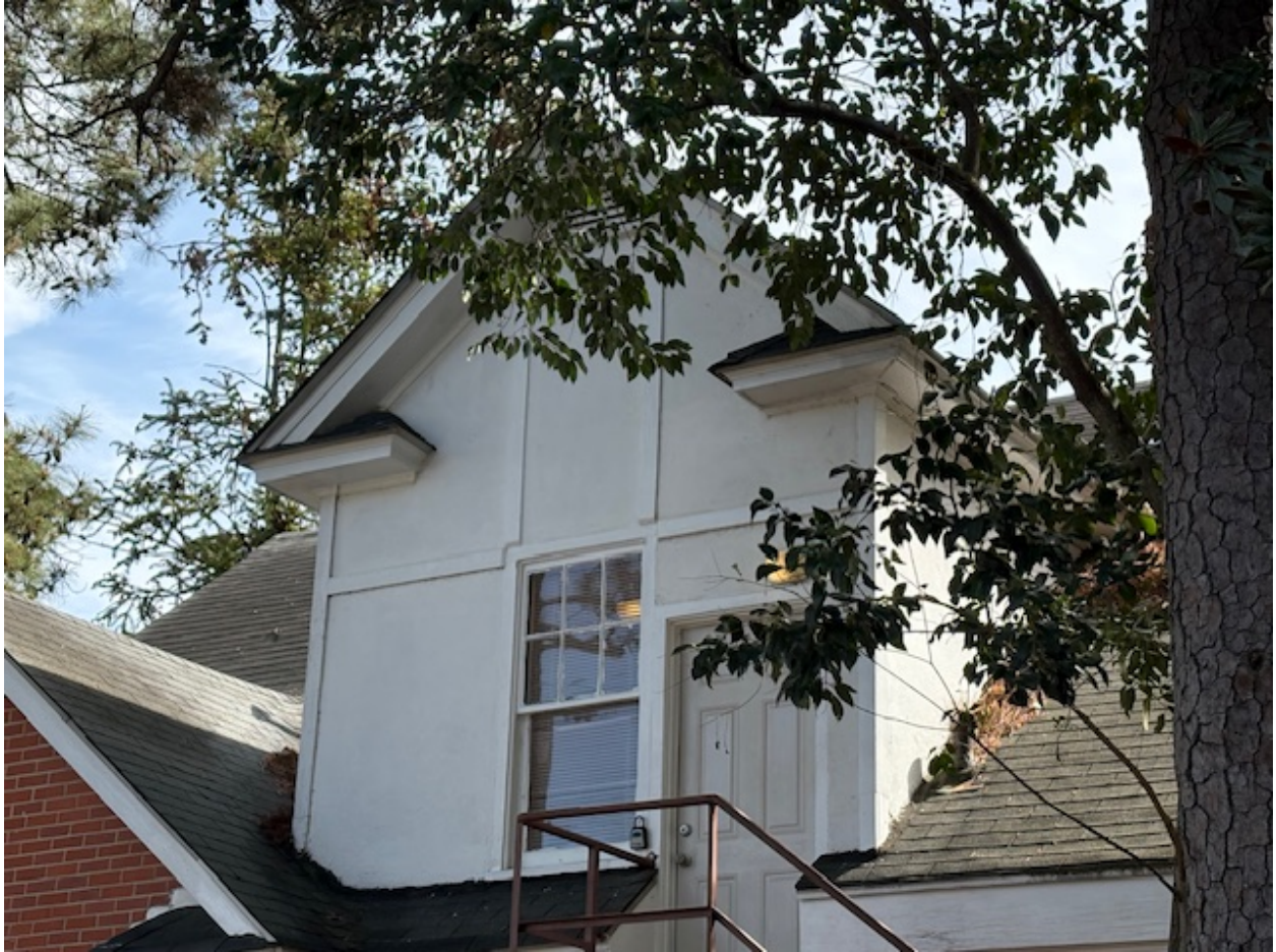
Closeup of current finish on gables.
